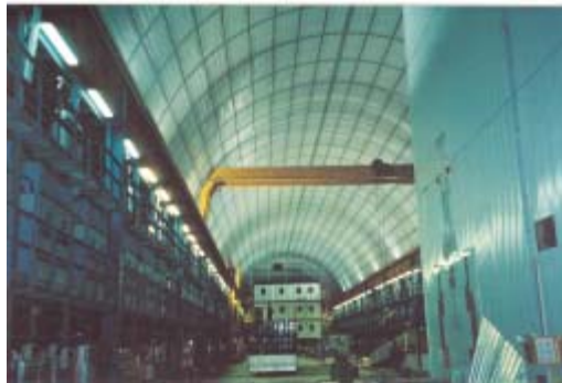
Paraffin oil tanks in one of the main underground experiment halls of the Gran Sasso National Laboratory in central Italy
